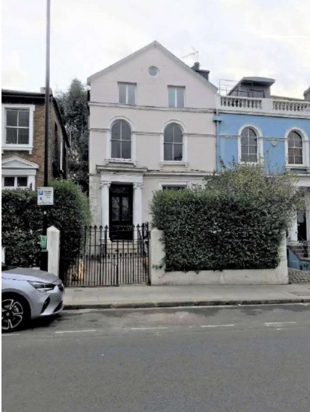
Photo of pre-existing front elevation
