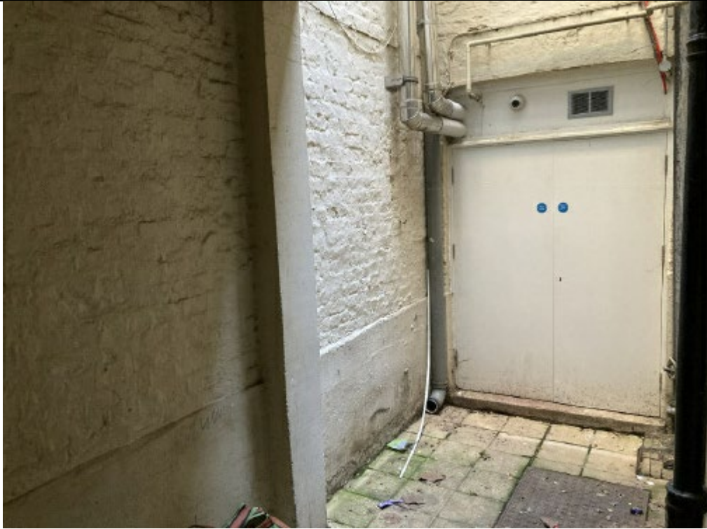
View within courtyard where the 5 air source heat pumps will be located
