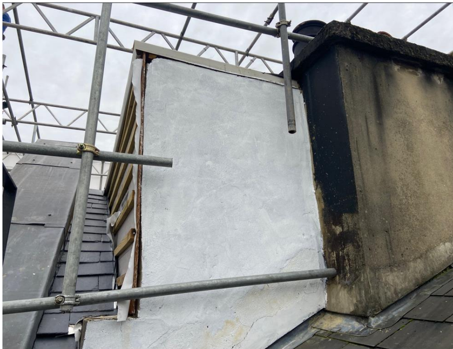
Photo of dormer to west side dated 16 November 2023
