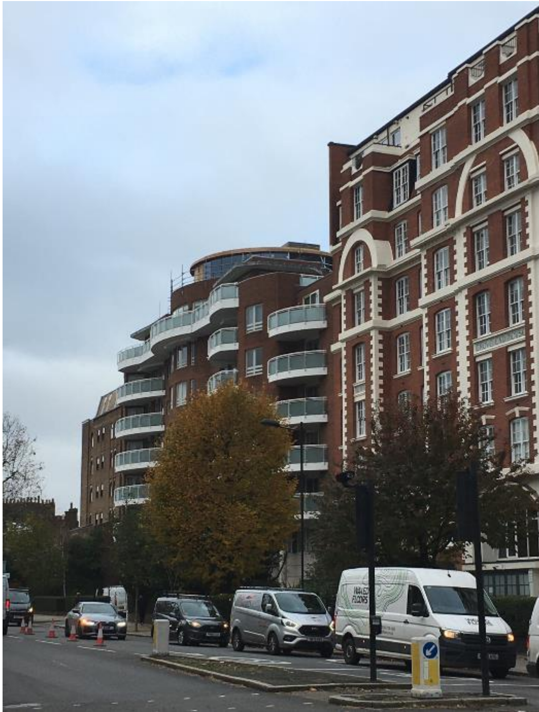
Front Elevation – roof extension as approved under 21/03579/FULL partially built.
